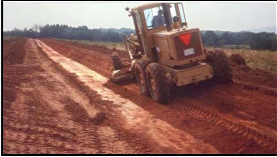
**Soil excavated when forming the channel is used to construct the berm**
