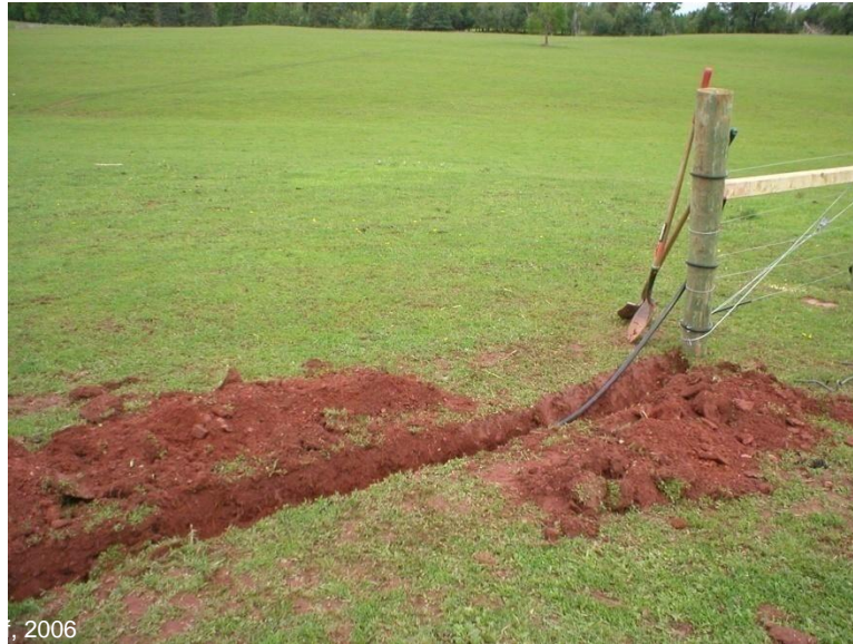
Figure 3.5 Wire run through water hose underneath gate
