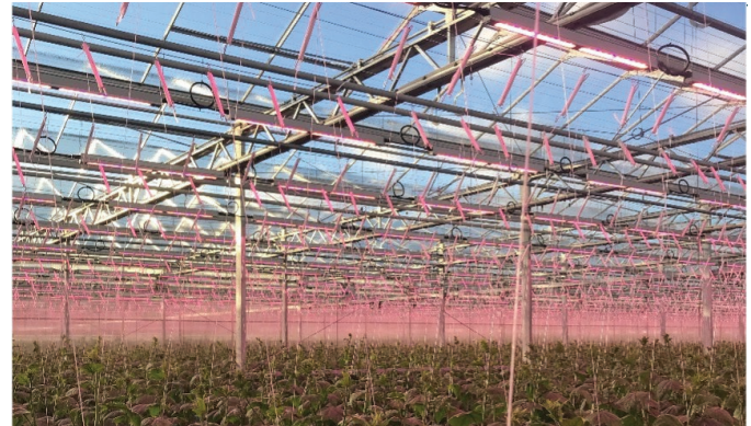
Figure 4. A supplemental LED lighting system implemented in a cucumber crop. Notice the thin profile of the lights, which reduces the shadows cast on the crop from the overhead light. Compared to the traditional fixtures, we see a higher density of lights required to provide adequate energy to the crop. Photo credit: Talia Plaskett, Perennia
