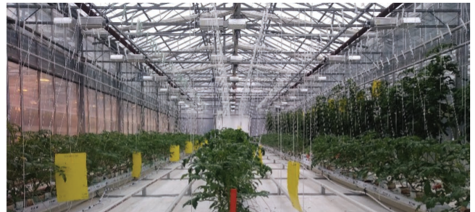
Figure 2. Here is an example of a producer that has chosen to implement supplemental lighting. While most of the light will come through the glass ceiling, the lights will be there to provide the plants with energy through the winter months. Photo credit: Talia Plaskett, Perennia
