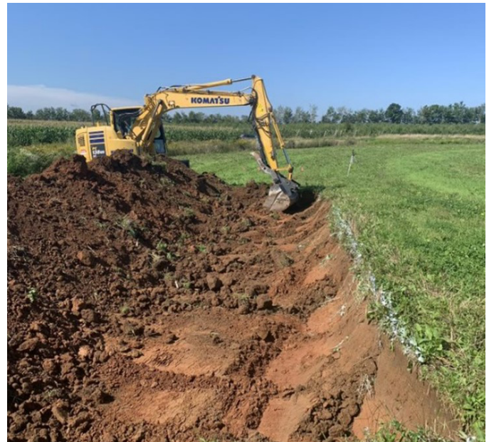
Figure 16: Step one of above-ground burial: dig a shallow trench
