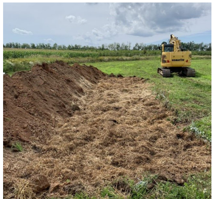
Figure 17: Step two of above-ground burial: place a 20cm layer of carbon material
