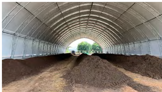
Figure 7: Windrow compost piles on concrete pad
