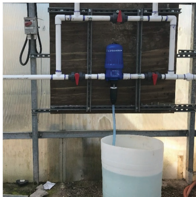
Figure 8. An image of a dosatron, used for injecting set amounts of concentrated nutrient solution into the irrigation water.
